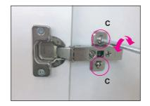
C on each mount plate, adjust door height by moving door up or down, then retighten C screws
